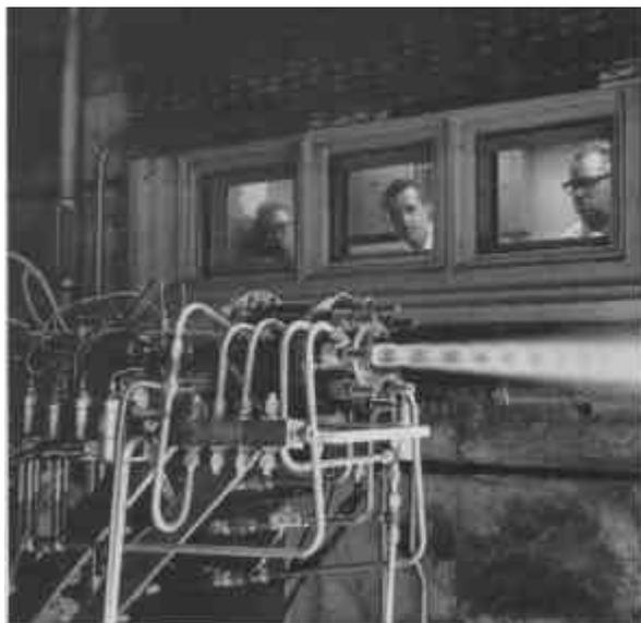
**Figure 8. Test Firing of Earliest TRW Pintle Injector Engine, a Water-Cooled MIRA 500**
